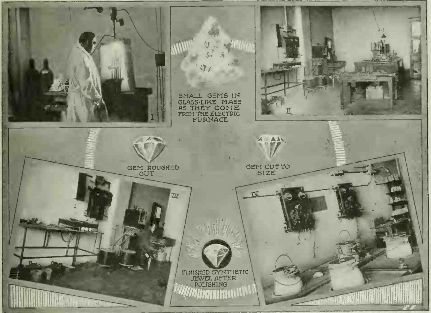
Manufacturing Precious Stones in the Electric Furnace: 1—Dr. Maurice Aisen at Work Making a Synthetic Gem in the Fierce Heat of the Electric Arc—the Greatest Heat Known to Science. 2—One View of the "Gem Making" Laboratory. 3—Another View of Dr. Aisen's Workshop, and 4—a Close-Up Glimpse of a "Battery" of Electric Furnaces in Which Rubies and Emeralds Are Turned Out by the Hundred for the Jewelry and Allied Trades. The Evolution of These Synthetic Jewels Is Illustrated by the Small Border Views. They are "Roughed Out," Ground and Polished the Same as Regular Gems. Diamonds Have Been Made in the Electric Furnace, But the Synthetic Diamond Cannot Be Manufactured Economically Just Yet.
